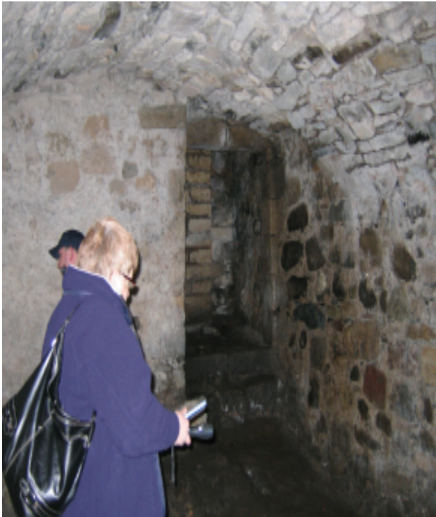
Lower floor of the Elphinstone Tower.
